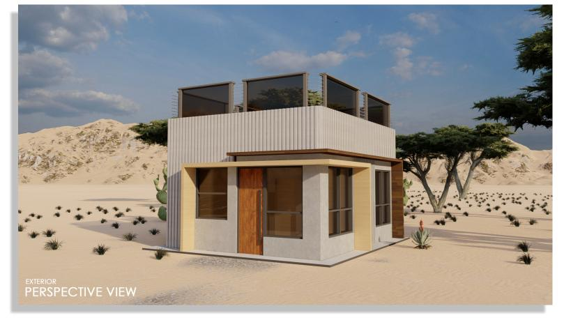
COAST ADU walls are sealed with precut insulation board. Installed outside boards, prewired and plumbed steel frame. The ceiling strength of the same MGO boards will hold Solar Panels on the flat rooftop.
